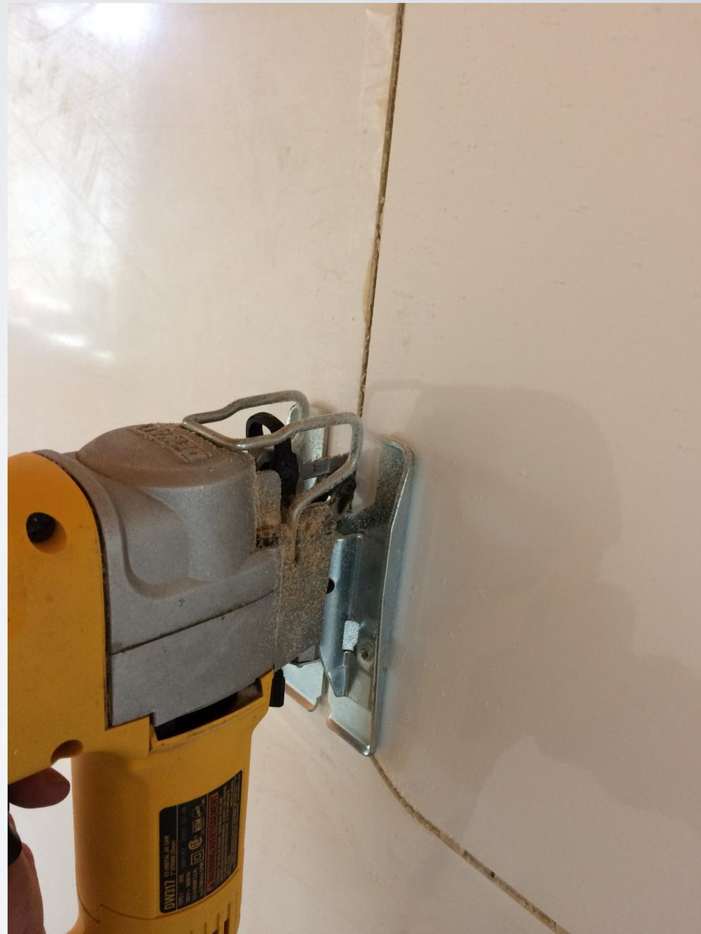
Use included metal clamps and screws to secure (dry fit) door frame. These clips can be removed after adhesive is cured.
