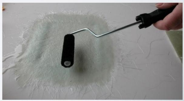
After resin is cured, fill surface with automotive micro filler. Sand and fill till smooth and even. After this stage you can apply automotive finish to blend repaired area in with surrounding.
