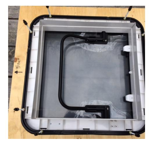
Place plywood jig on roof and trace the cutting line with permanent marker.
