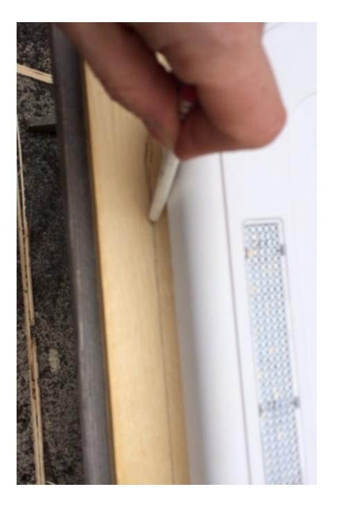
Create a second line 3/4" (19mm) on INSIDE of the original line. Cut along the inside line with Jigsaw
