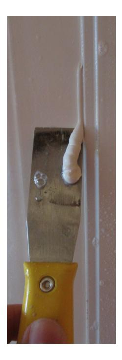
Push hatch into opening. Don't push too hard as you need 1/16 thickness of adhesive between roof and hatch to guarantee waterproofing.
