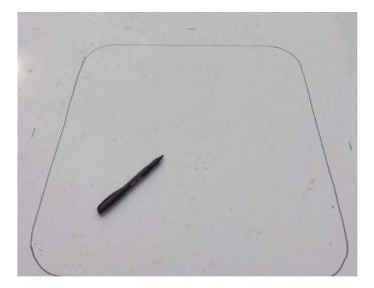
Use Metal blade for Jigsaw and cut along the marker line. Remove roofing material.
